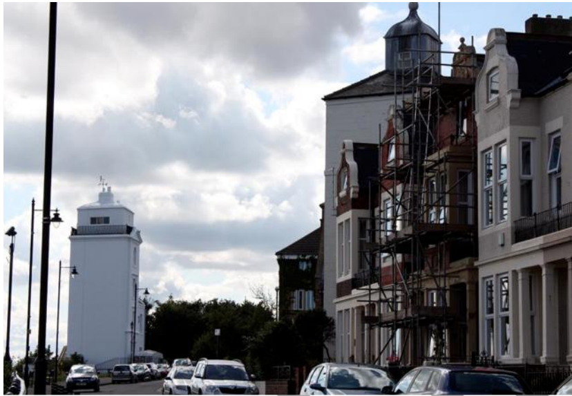
High Light and Trinity Building
