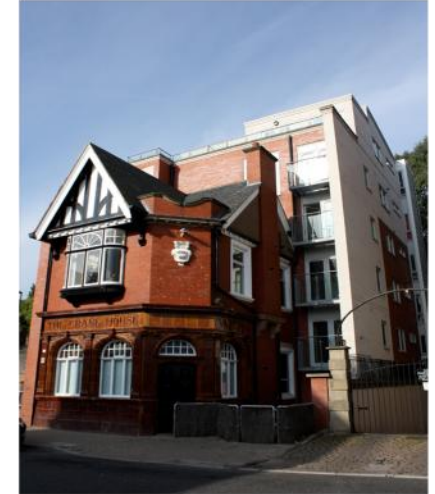
Chain Locker Apartments
