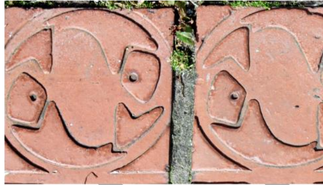
Decorative street paving tiles
