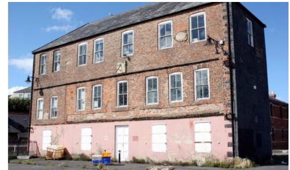
The former Old Low Light currently under refurbishment
