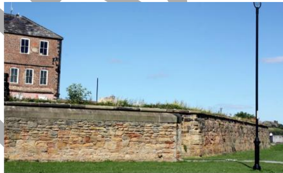
A section of wall at Clifford's Fort
