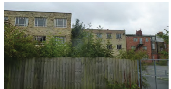
Boxy flat-roofed offshots in non-matching materials, behind Northumberland Square
