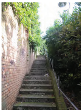
Steps to Liddell Street feel quite overgrown and claustrophobic
