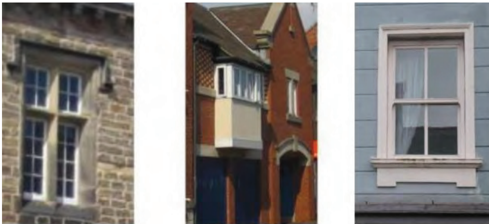
(1) Window incorporating transom, mullion and lintel (2) Oriel window (3) Window with apron and horns
