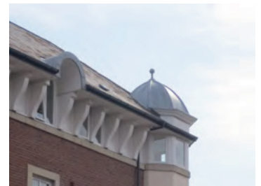
Exaggerated timber brackets and zinc dome at No. 111 Howard Street
