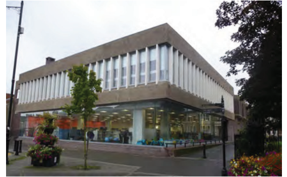
The columns of the Library straddle the Metro tunnel beneath
