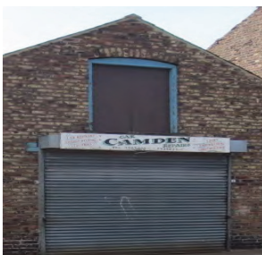
Converted stables, North Zone
