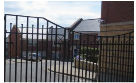
Apparent two storey height at Union Stairs, where the foundations are below in Liddell Street.
