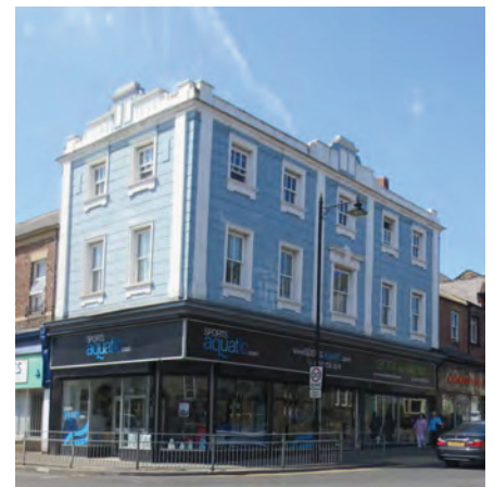
A modern shopfront with large windows and fascia harms the building's character
