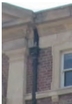
Decorative gutters, Business Centre
