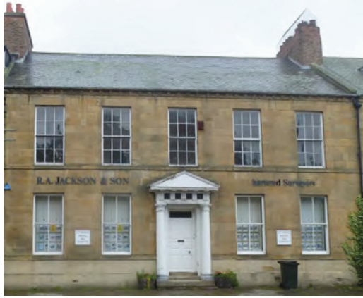
Timber vertical sliding sash windows
