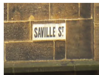
Features, such as historic nameplates, should be retained
