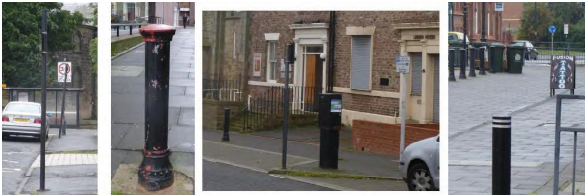
Copious amounts of other street furniture, some unfortunately sited, much of it uncoordinated and in need of repair
