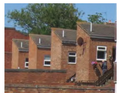
Offshots, Stephenson Street
