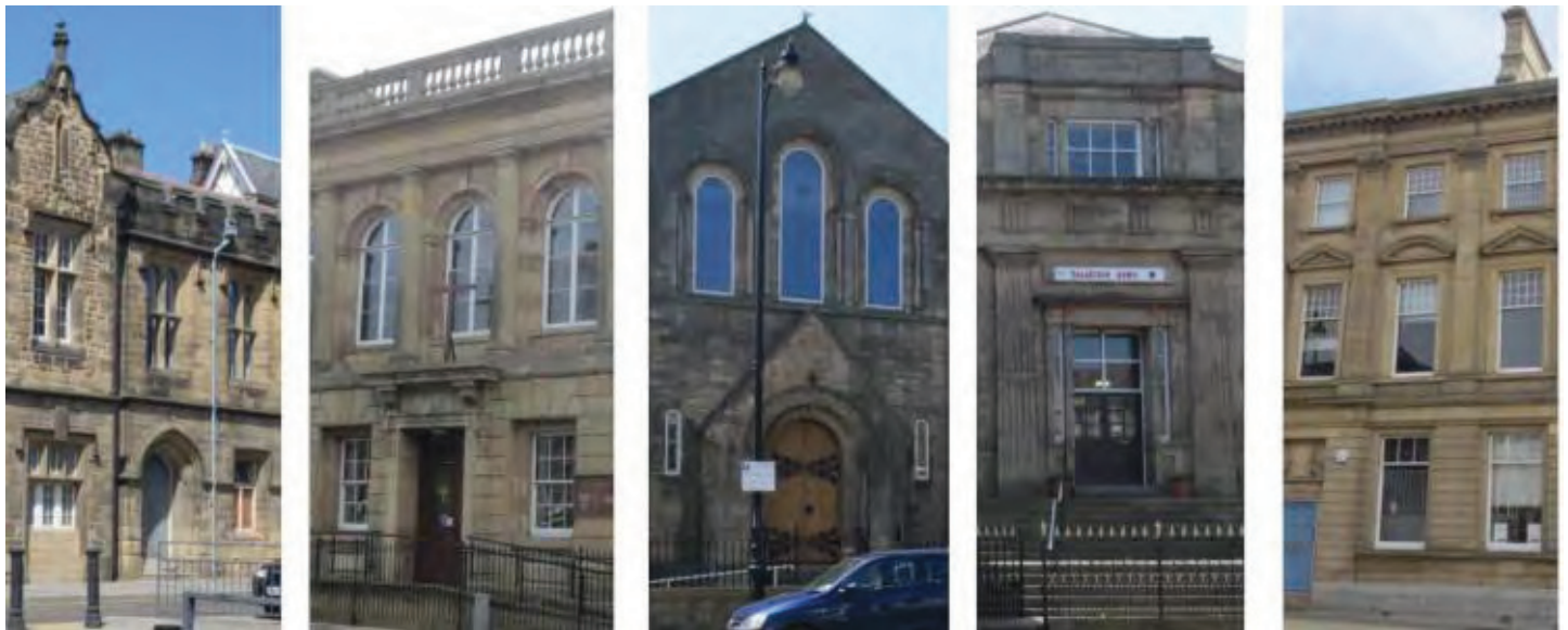
Worked sandstone expertly used to create architectural styles: Tudor gothic, Palladian, Romanesque, Greek Doric and Italianate
