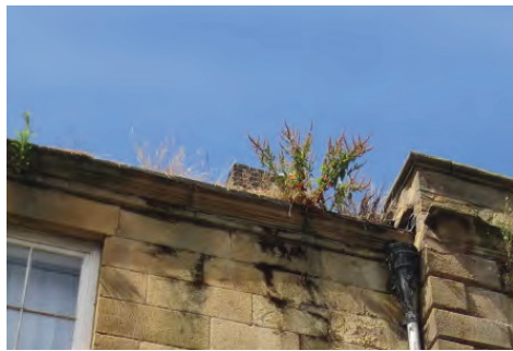
Neglect is unfortunately beginning to show in some parts of the conservation area
