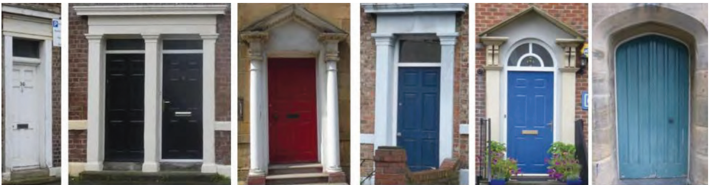
Typical doors and surrounds - North, Central and South Zones
