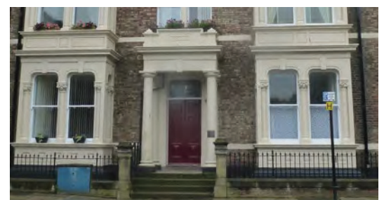
The west side of the Square with stone gate piers, railings and stone plinths
