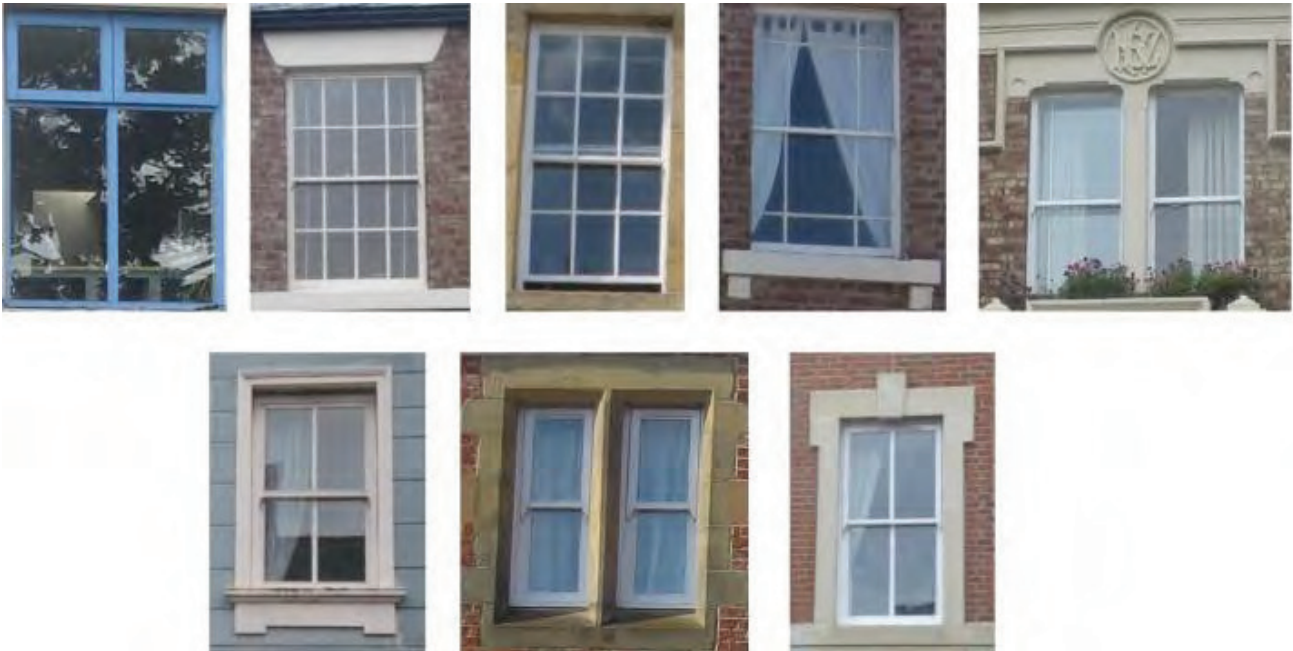
North and Central Zone (above). Typical replica windows - South Zone (below)
