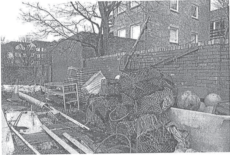
Sycamore tree abutting boundary wall and substation
